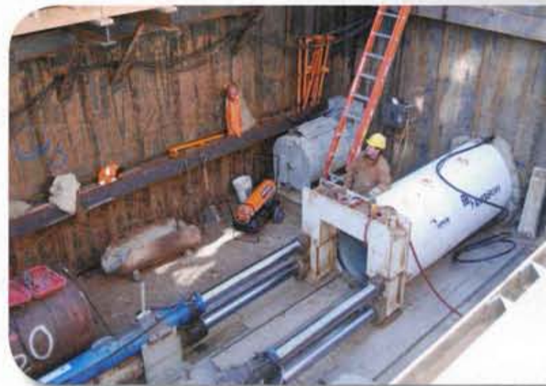
M&P Pipe Jacking uses four 200-ton Rogers hydraulic jacks to push 36-inch Hanson RCP sewer on C.J. Fucci Construction's $12-million sewer separation project in New Haven.
